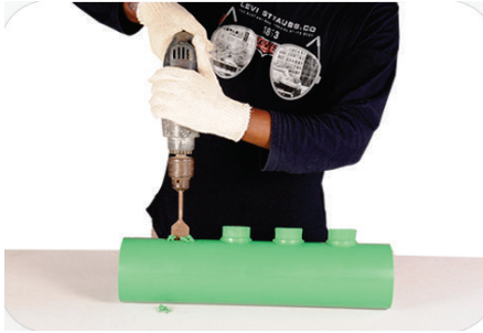
Drill with Proper Diameter and Make Correct ID Hole
